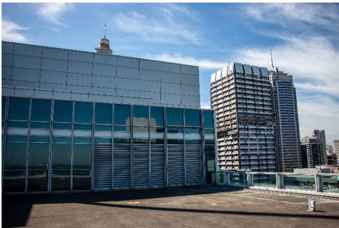
Figure 11 View from the existing roof looking east
