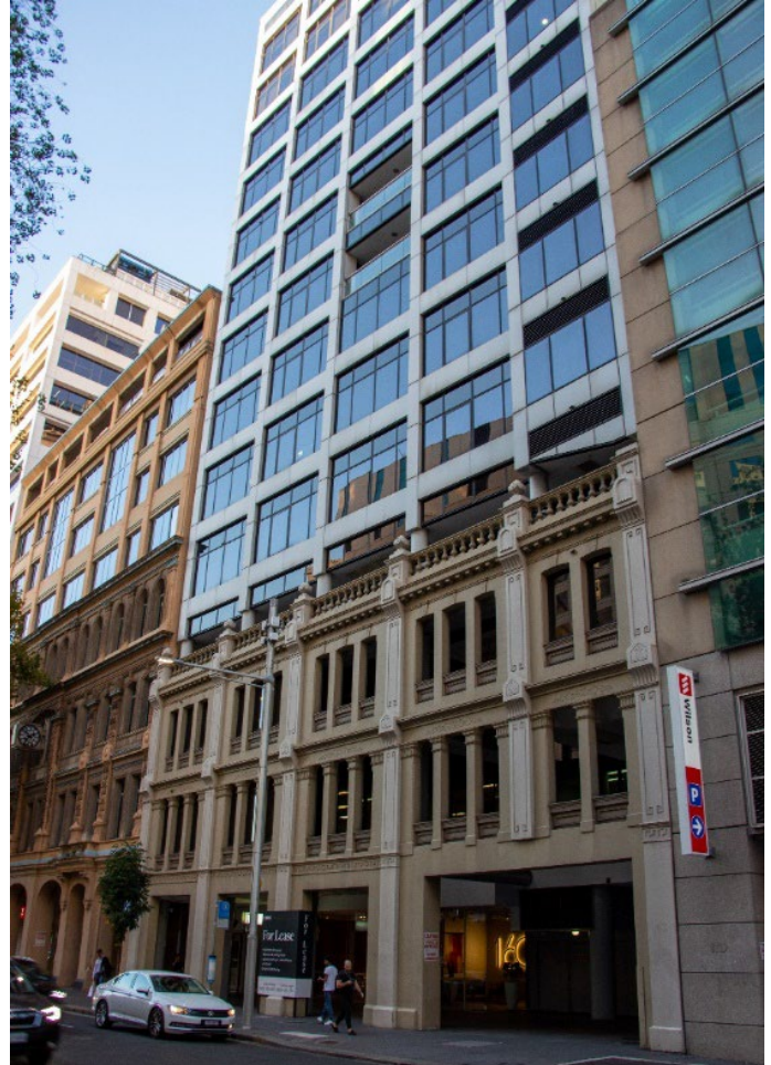
Figure 18 View along Sussex Street to the north
